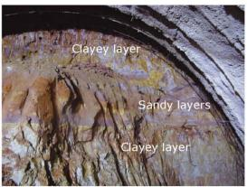
Fig. 10.4.2. Heterogeneous soils
